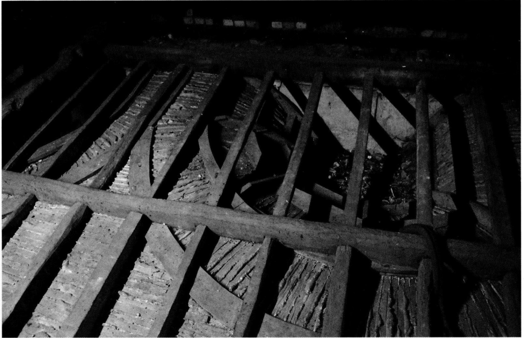
Fig. 12 The chapel, the lath and plaster construction of the ceiling Photograph, M. Saunders
